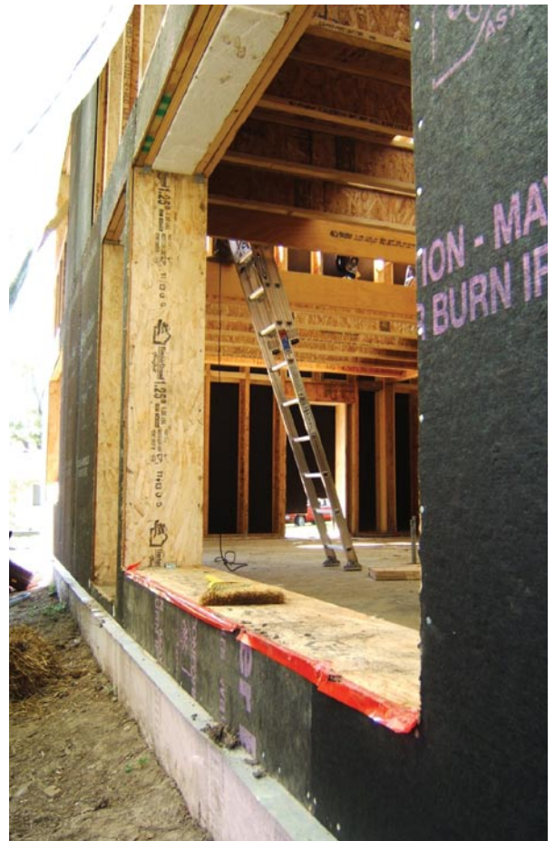
The Fairview House’s well-sealed 14-inch thick walls make for a very low energy home and very affordable energy bills.
