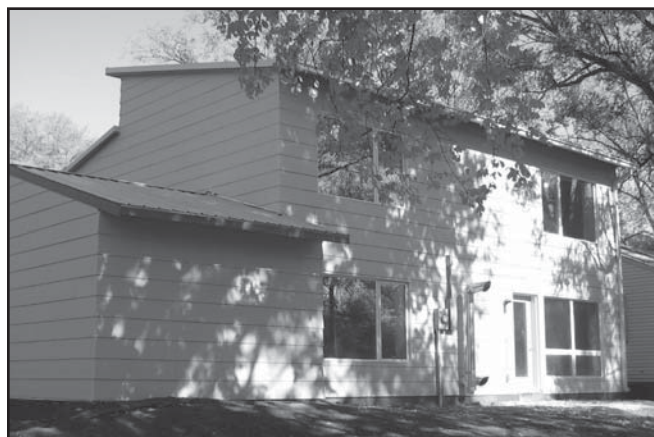
Figure 1. Most of the windows at the second Passivhaus in Urbana, Illinois, face south. This photo shows the ventilation system's intake and exhaust ducts.
